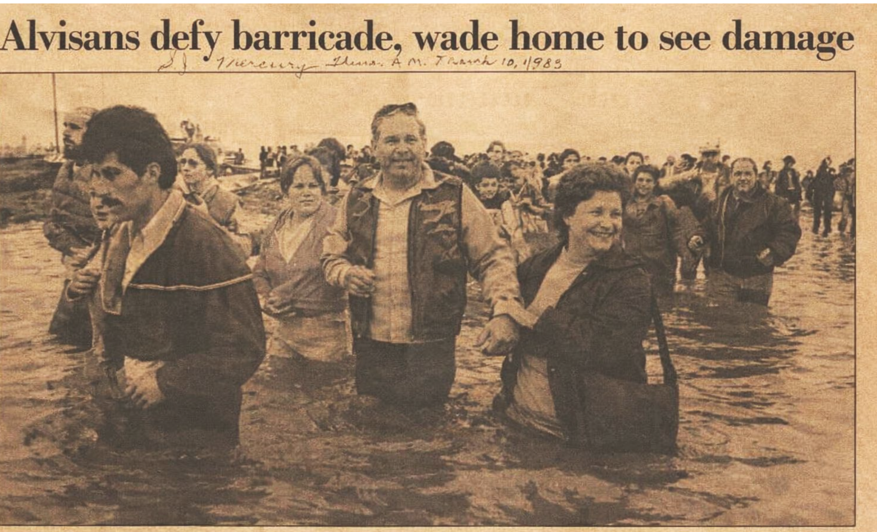
Figure 1. Major flooding event in Alviso in 1983. Photo sourced from San Jose Mercury.
